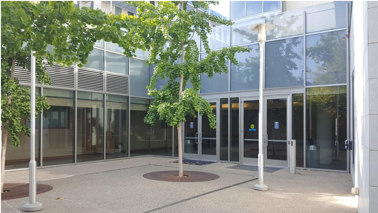
Below-ground courtyard with entrances to meeting area.
